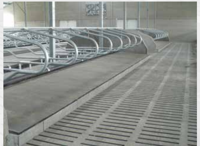
A finished project. Here with the cubicle beds on the slats.
